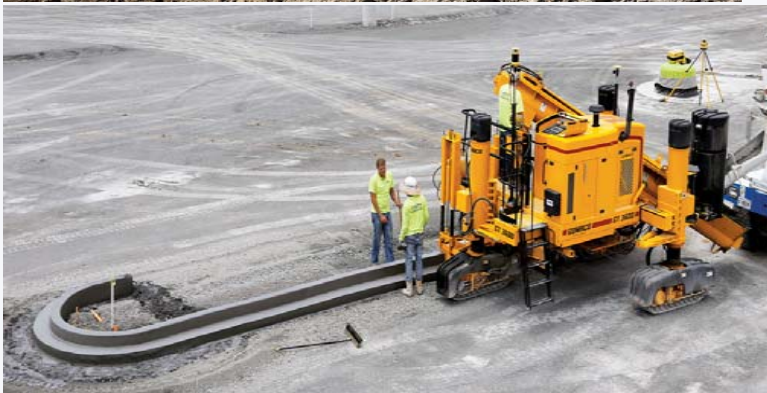
3D Machine Control Excavator, Concrete Curbing Paver
